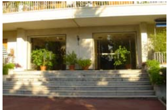
Entrance to apartments from Garden
