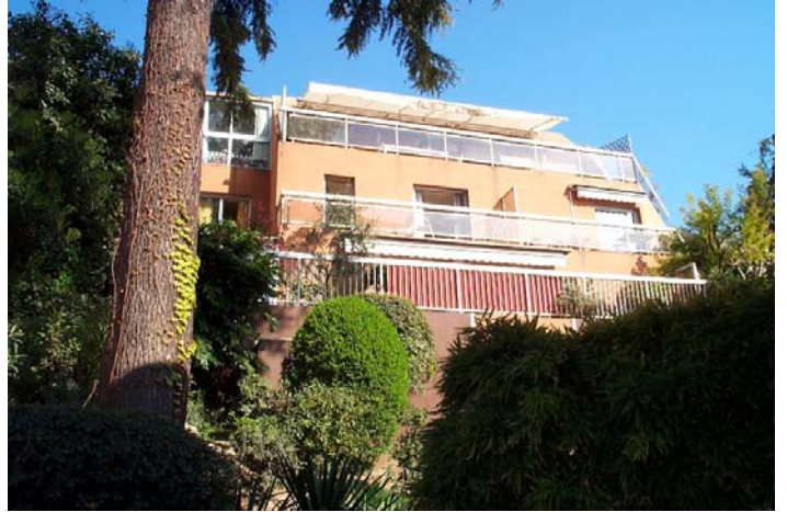
The apartments set into the hillside
